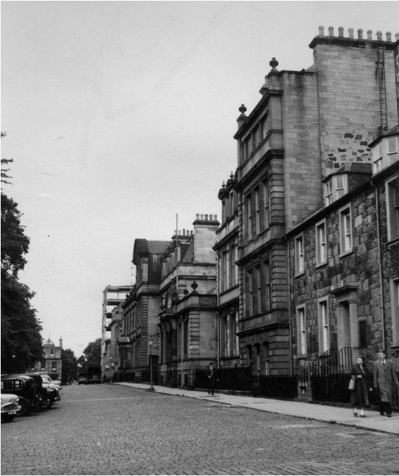
Fig. 3. North George Square, c. 1959. On the right are Nos 1 and 2, followed by George Watson's Ladies College, on the site of Nos 3–7. Beyond is the portico of the Forestry building, on the site of Nos 8–10. At the far end can be seen the structural steelwork for the first phase of the Medical Extension. ( Edinburgh University, EU, Fenton Collection. )
