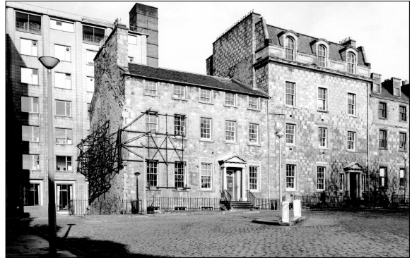
Fig. 24. Nos 13 and 14 George Square before demolition in 1976. No. 15 has already been removed, and scaffolding supports the gable wall. Part of the Pathology Building can be seen behind. (Courtesy of Andrew Fraser.)
