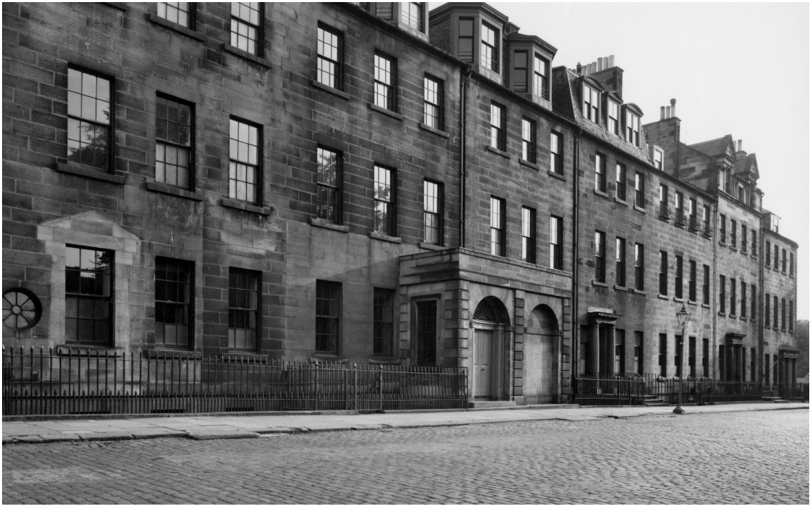
Fig. 4. The west half of the south side of George Square, showing how much the façades of Nos 30–38 had been altered by 1959. On the right, the doorway of No. 32 was removed when it was incorporated into Masson Hall. The doorway to Cowan House (No. 35) shares a porch with No. 34, now blocked. On the left, the portico of No. 36 was removed when the door was converted to a window. All the buildings have also been extended upwards in one way or another. ( EU, Fenton Collection. )
