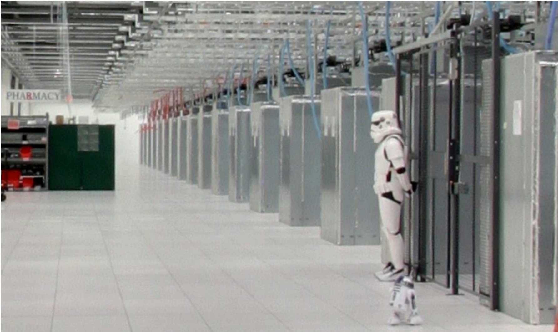
Google data center, Lenoir, North Carolina, US
