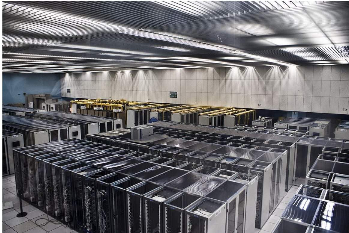
Server Farm at CERN
